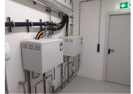
Water Preparation Unit (left) and Steam Generators (right)
